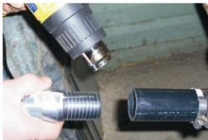
The ABS pipe has to be heated with a heat gun or hair dryer before the ABS will receive the galvanized nipple. Once inserted, the clamps should be tightened quickly while the ABS is soft.
