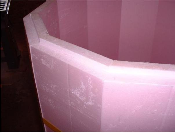
Assemble so that extended ends are all in the same position so that the top 4' sleeve overlaps the bottom 4' sleeve.
